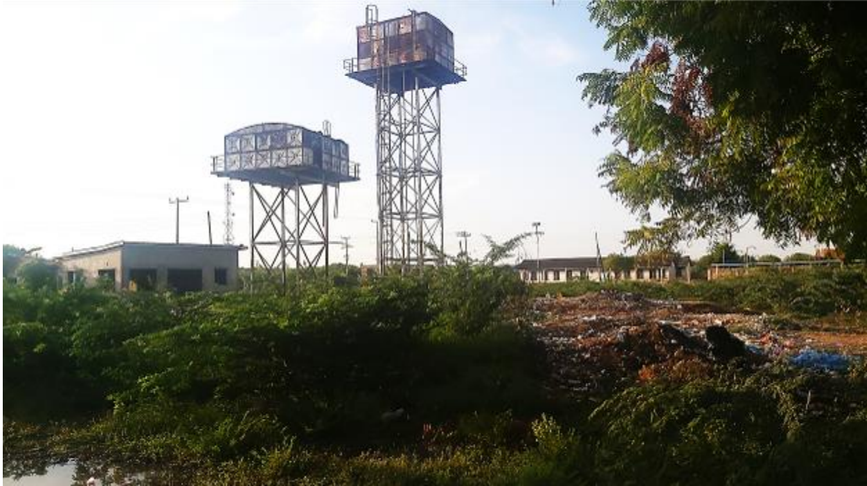
Figure 6: The elevated metallic water tank serving the hospital (Source: Field Work)
