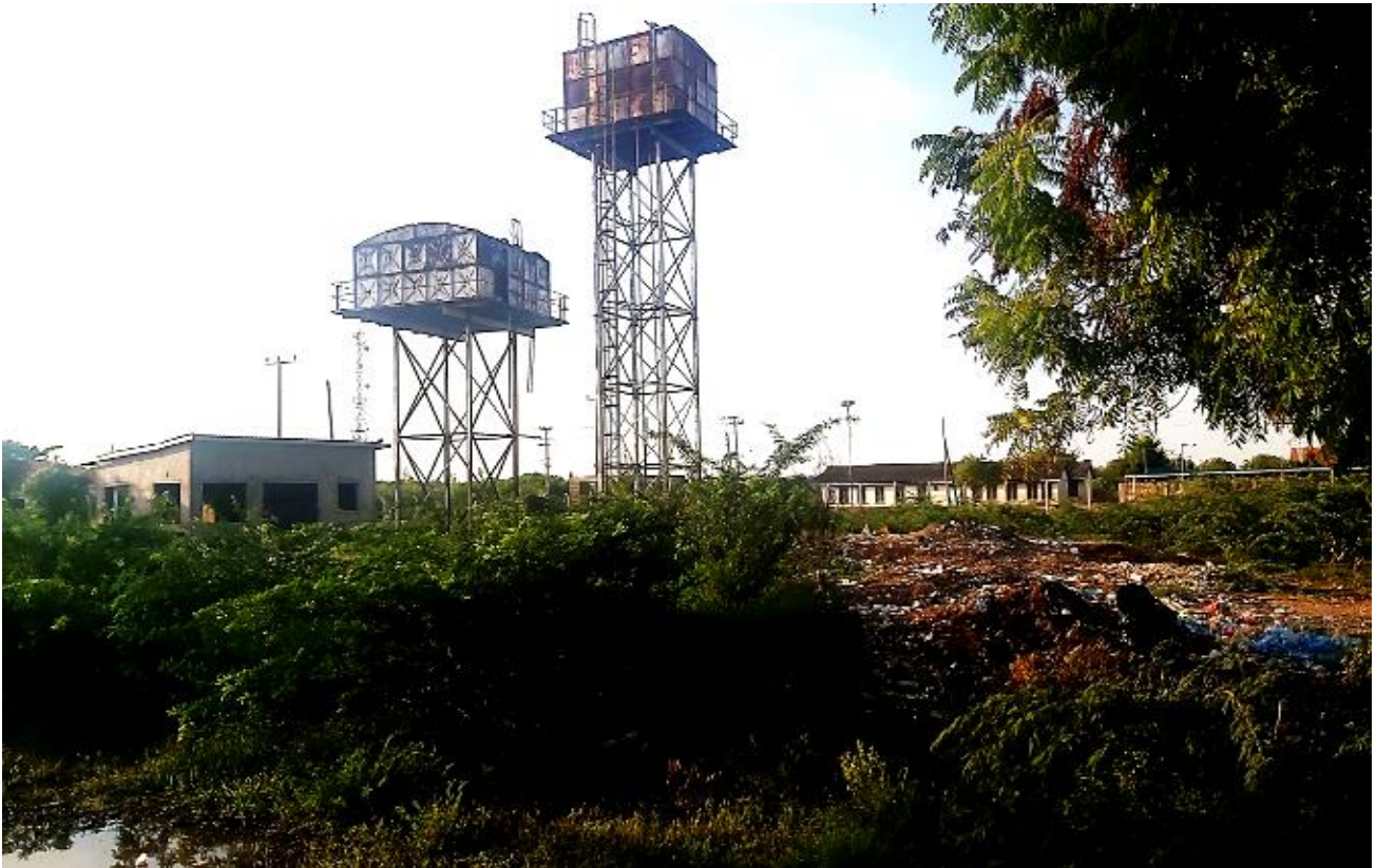
Figure 3: The project site showing the constructed structure to the far left and open HCW disposal site to the right (Source: Field work)
