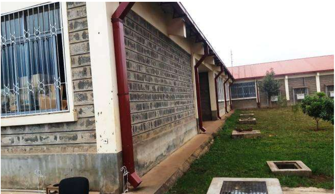
Figure 15: Some of the rain water gutters directing storm water on to open grounds (Source: Field work)
