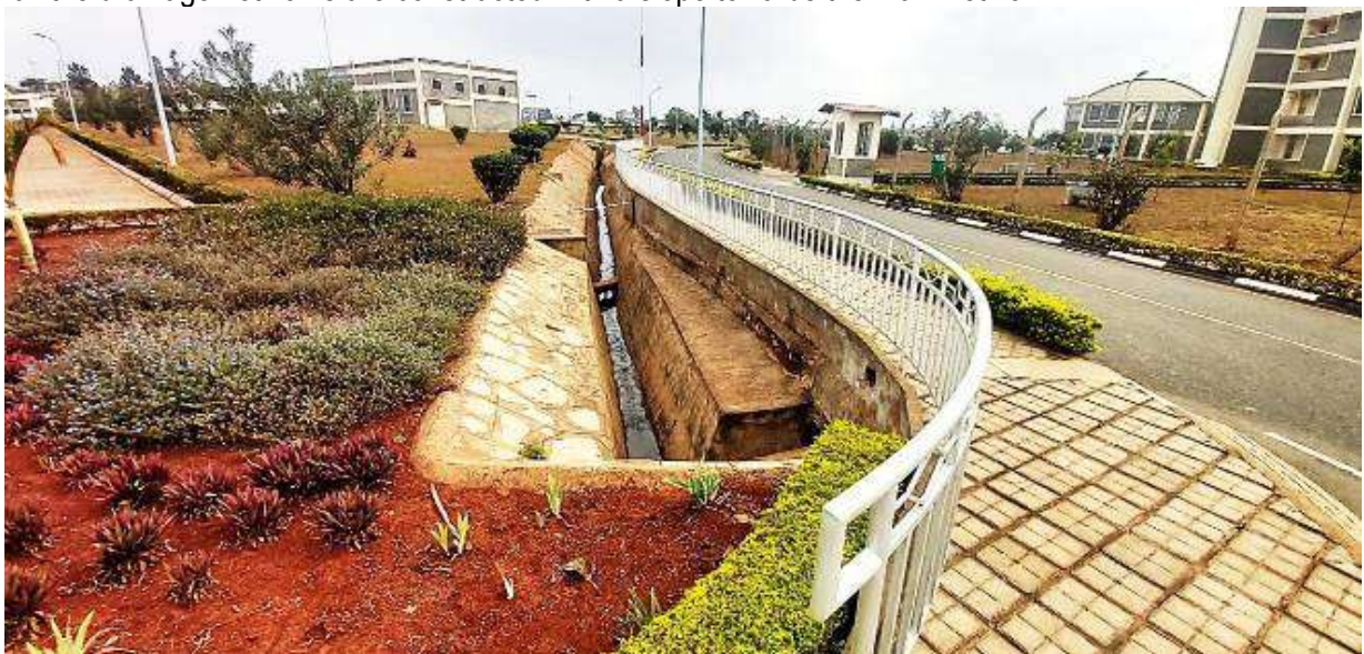
Figure 17: One of the well-constructed drainage channel within the hospital compound (Source: Field work)
