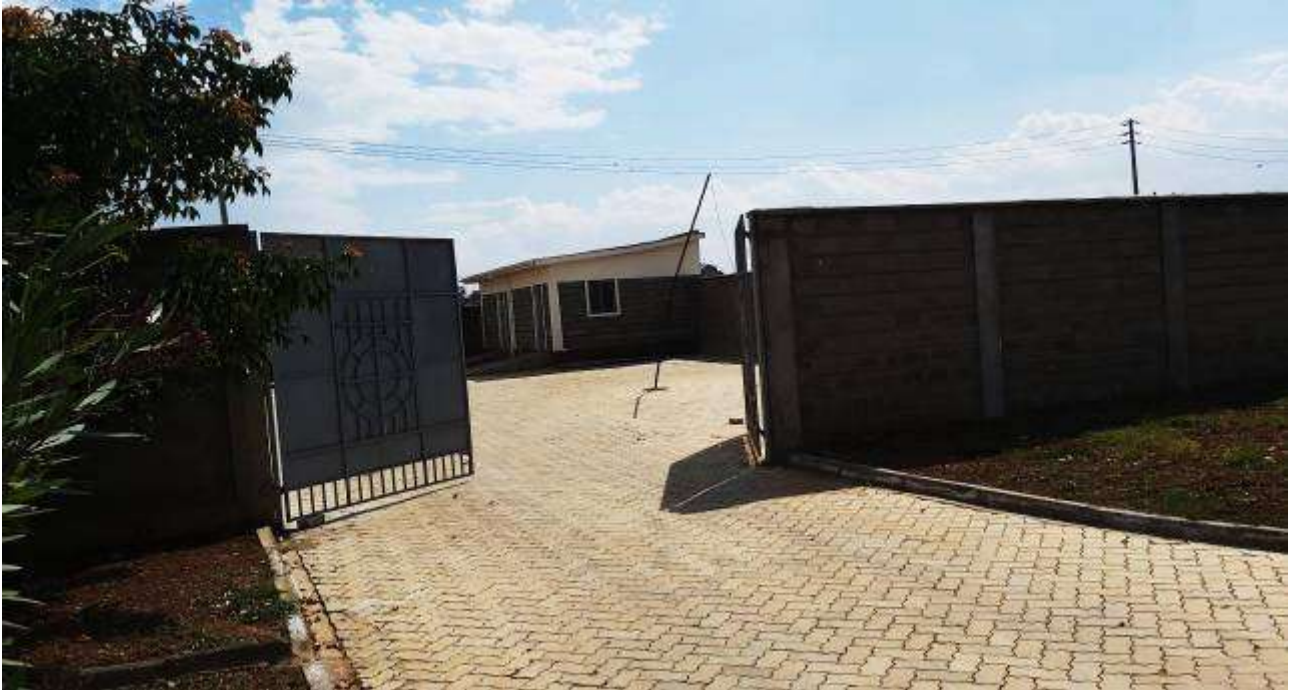
Figure 22: The rooms next to the MWTI shelter that could be converted to operator's office and store area (Source: Field work)
