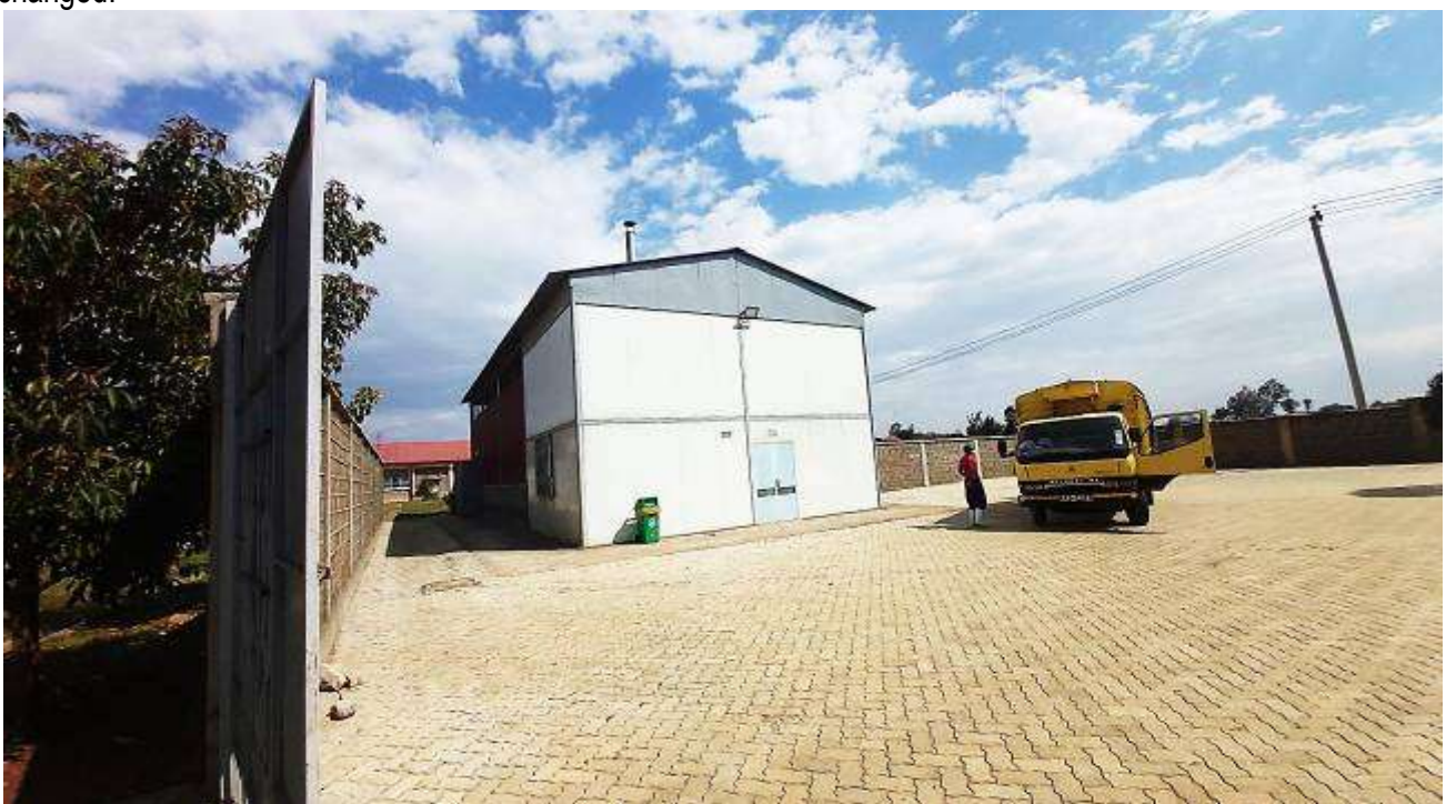
Figure 21: The already paved waste management area around the MWTI area (Source: Field Work)
