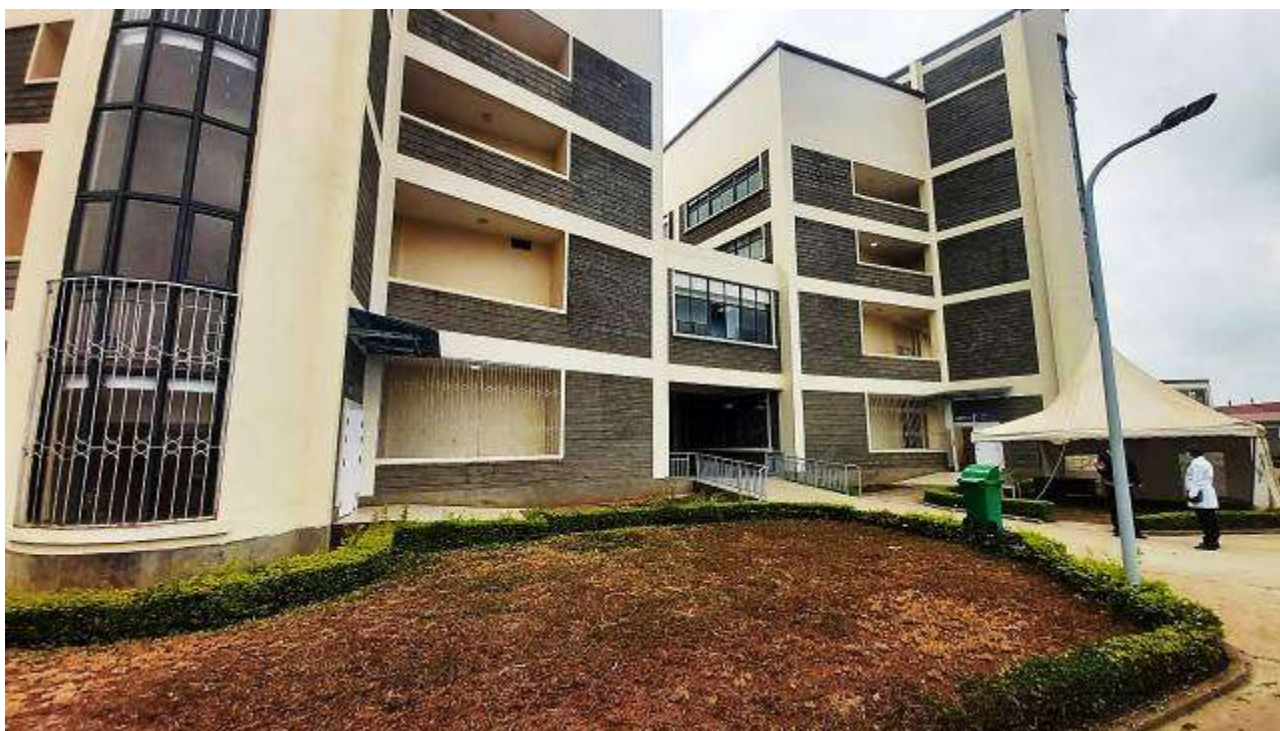
Figure 1: The block housing the wards earmarked for renovation/modifications (Source: Field Work)
