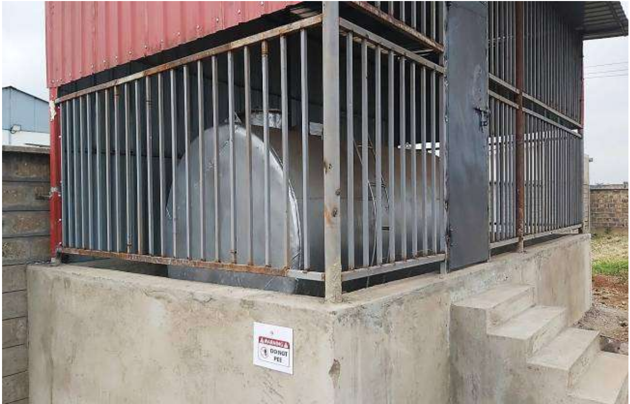
Figure 5: The 10, 000litres diesel storage metallic tank outside the MWTI shelter (Source: field work)
